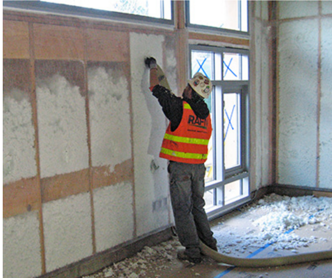
Blown-in cellulose insulation
